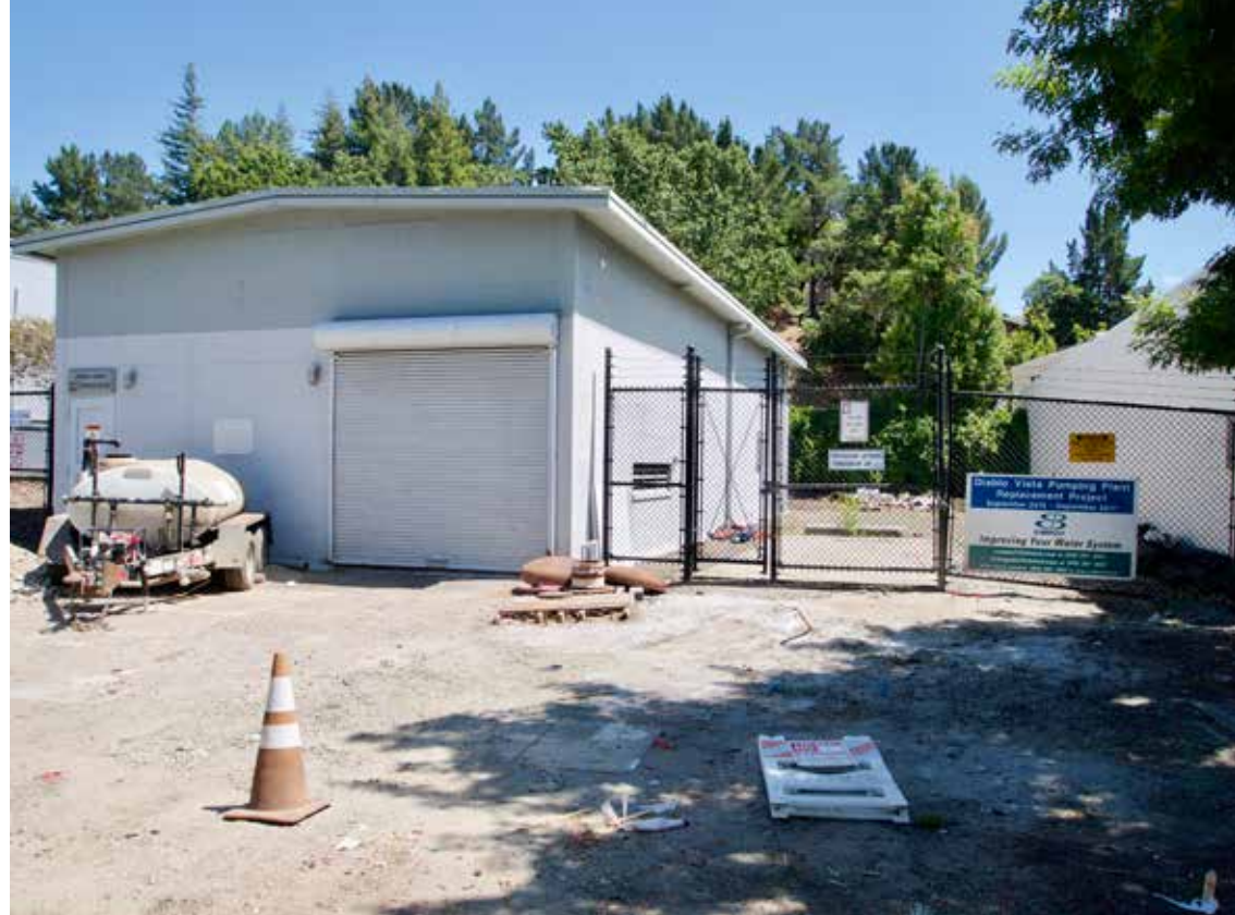
Demolition will soon begin on the old pumping plant next to Ace Hardware to make space for a new parking lot. Photo Pippa Fisher
